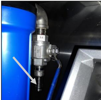
Figure 3: Inlet valve and hose barb.
